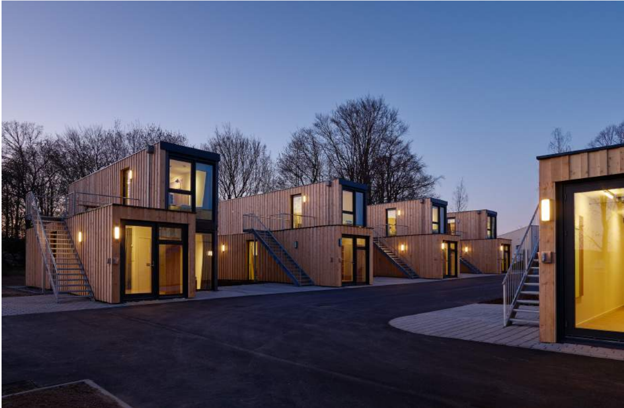
21 container modules from Containerwerk have been used for the first temporary living quarter created by MAX Wertheim GmbH in Wertheim, Baden-Württemberg.
