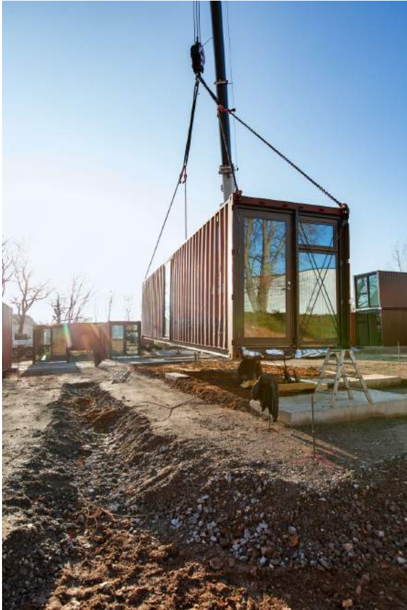
Strip foundations are sufficient. Completely sealing the ground is therefore avoided.
